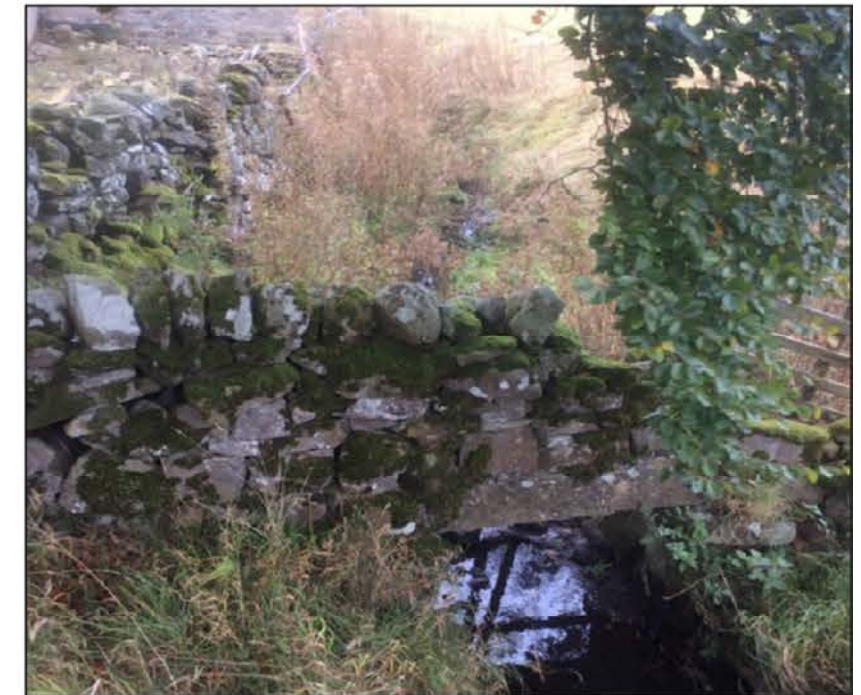
Photo Location 4: Facing downstream at culvert
