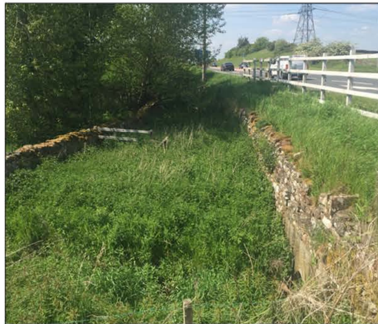
Photo Location 3: Right bank facing Watercourse
