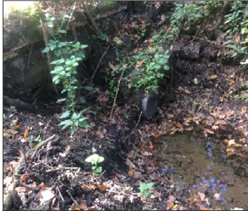
Photo Location 1: Left bank facing downstream at culvert
