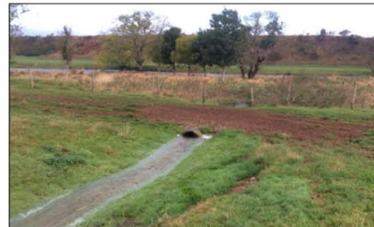
Photo Location 6: Right bank facing culvert downstream
