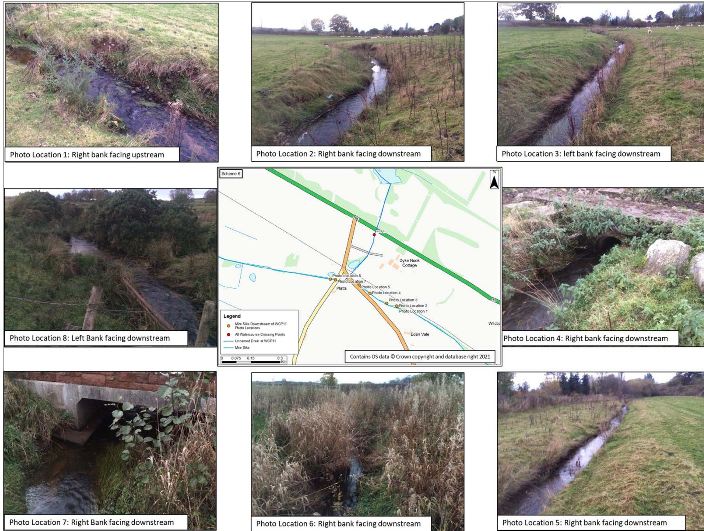
Plate A-34: Mire Sike Downstream of WCP11 site photograph locations
