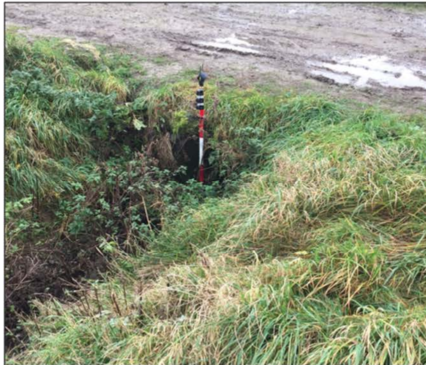
Photo Location 3: Facing upstream at culvert
