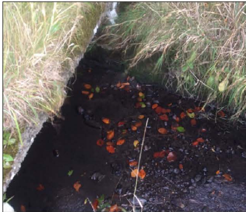
Photo Location 3: Facing upstream at culvert
