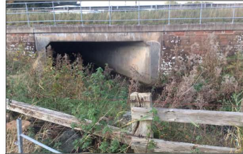
Photo Location 3: Culvert facing downstream
