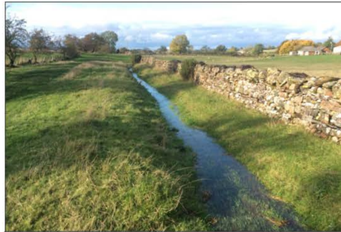
Photo Location 1: Left bank facing downstream
