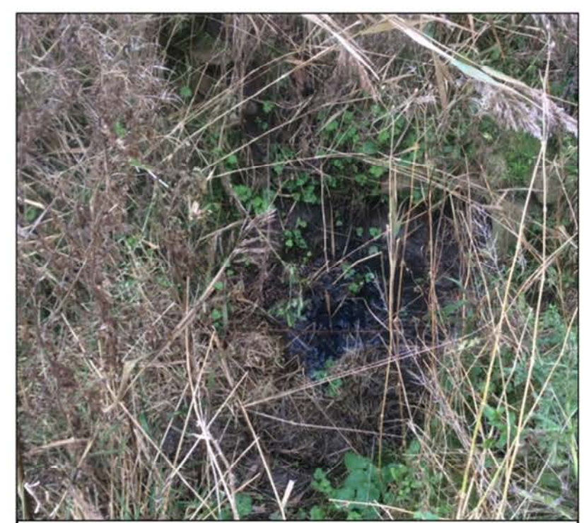
Photo Location 4: Left bank facing downstream
