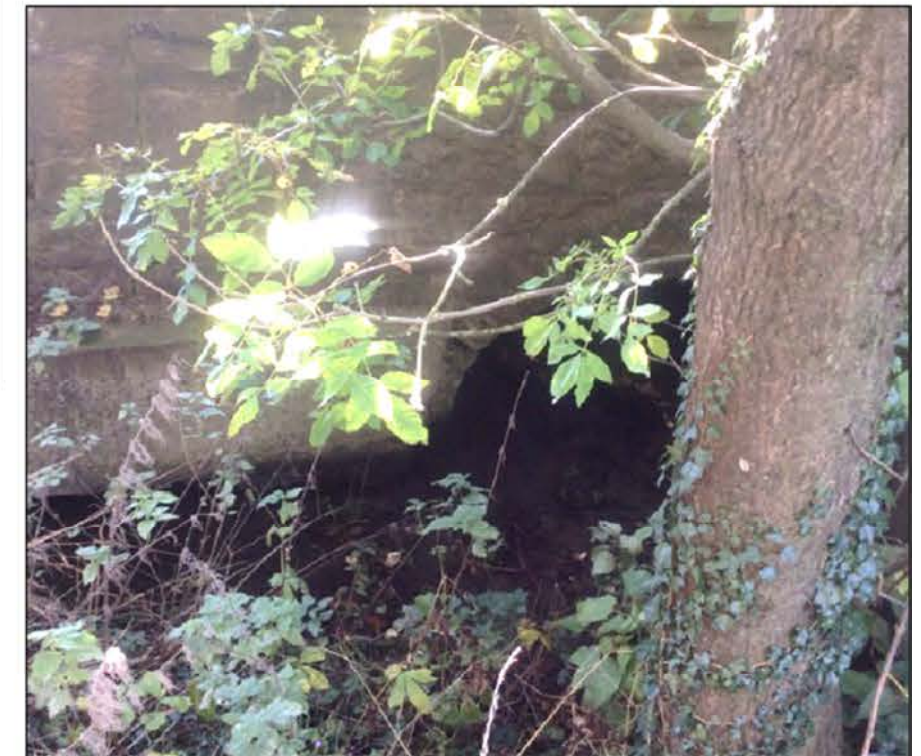
Photo Location 2: Right bank facing downstream culvert at A66
