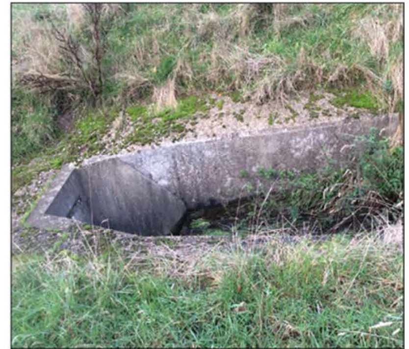
Photo Location 4: Left bank facing culvert at A66
