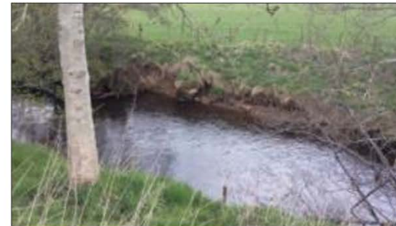
Photo Location 6: Left bank facing right bank
