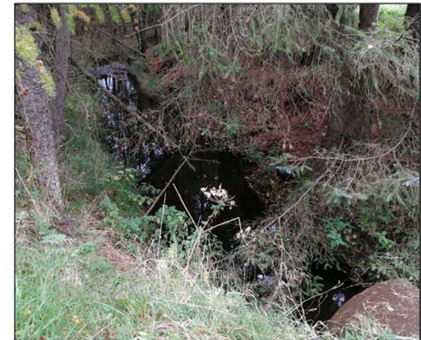
Photo Location 4: Left bank facing downstream at culvert
