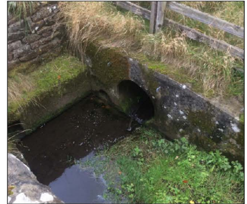
Photo Location 2: Left bank facing upstream at A66 culvert
